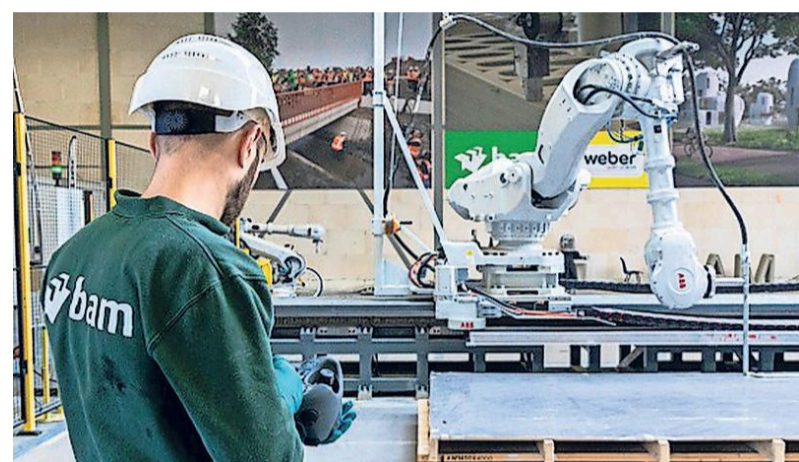
De 3D-betonprinter in werking.
