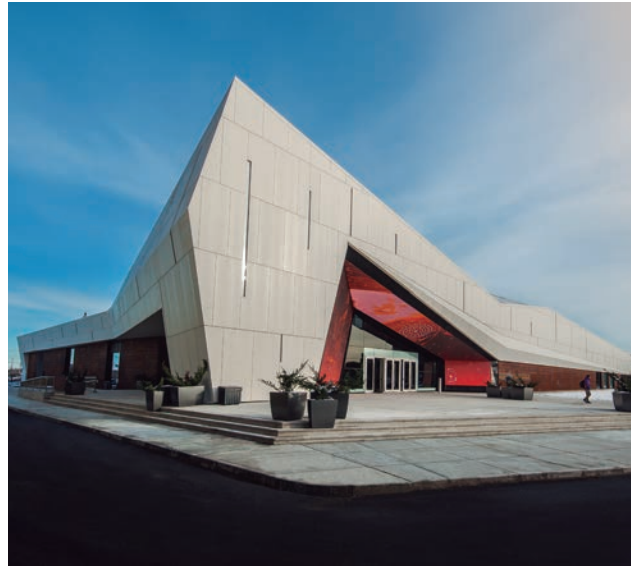
Canada Science & Technology Museum, Ottawa, Canada Designed by: NORR Limited Ottawa
